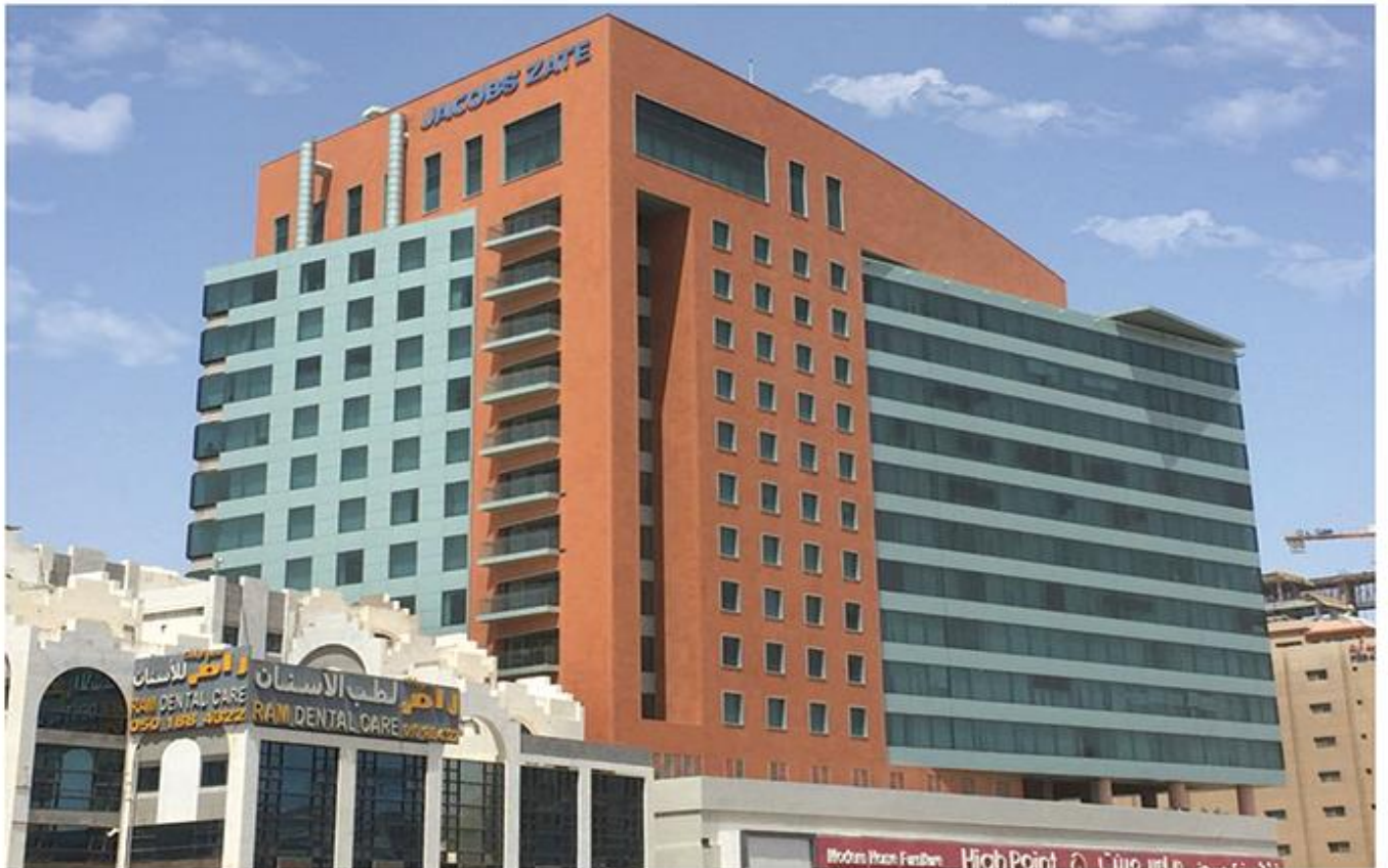
Alfamar Hotel Al Khobar Thermal Insulation & Waterproofing
