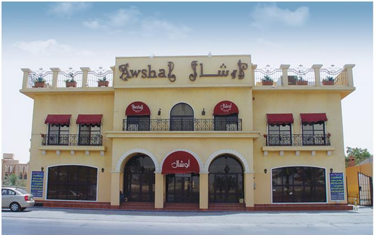
Awshal Restaurant Thermal Insulation & Waterproofing
