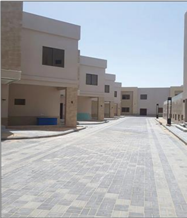
Alf Compound Al Khobar Complete Insulation System
