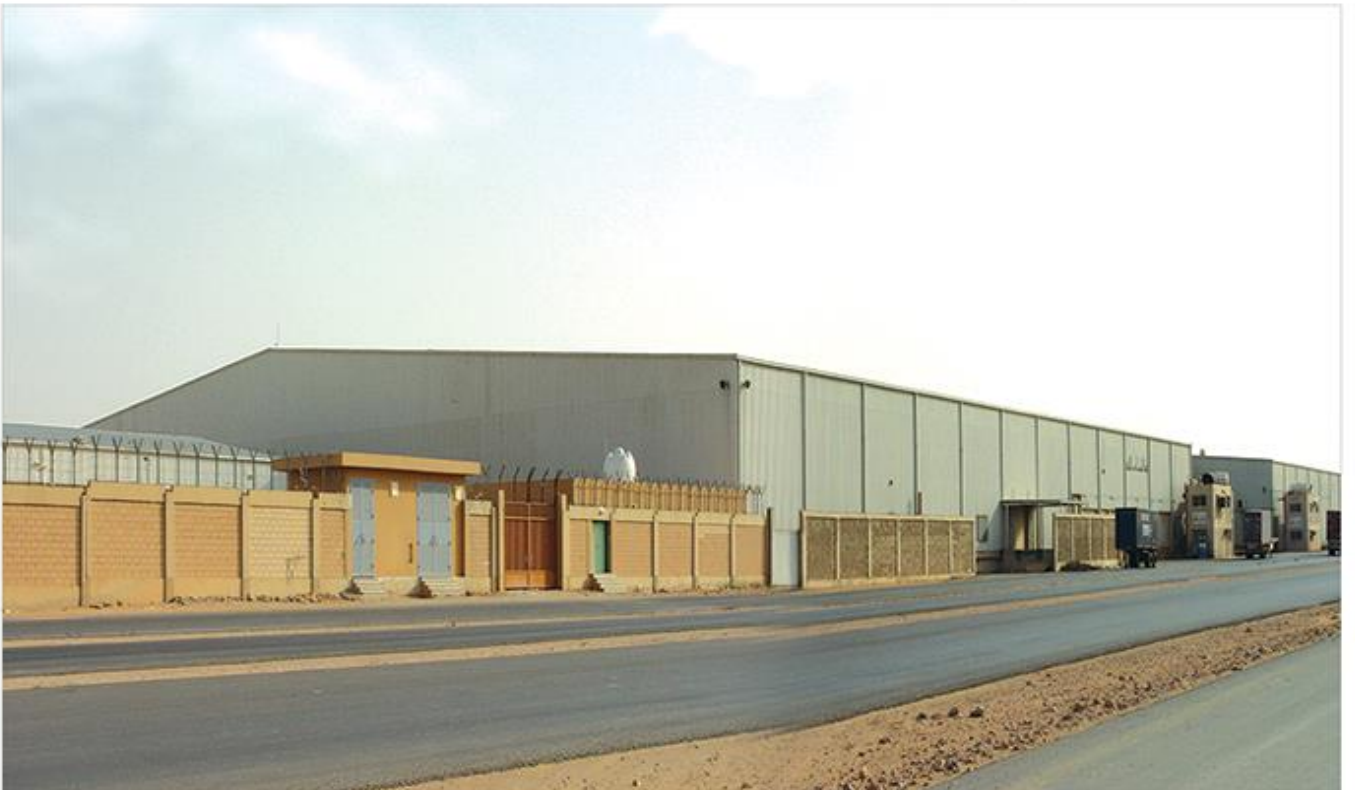
Jarir Bookstore Warehouse (34,000 sq.m.) Thermal Insulation & Waterproofing
