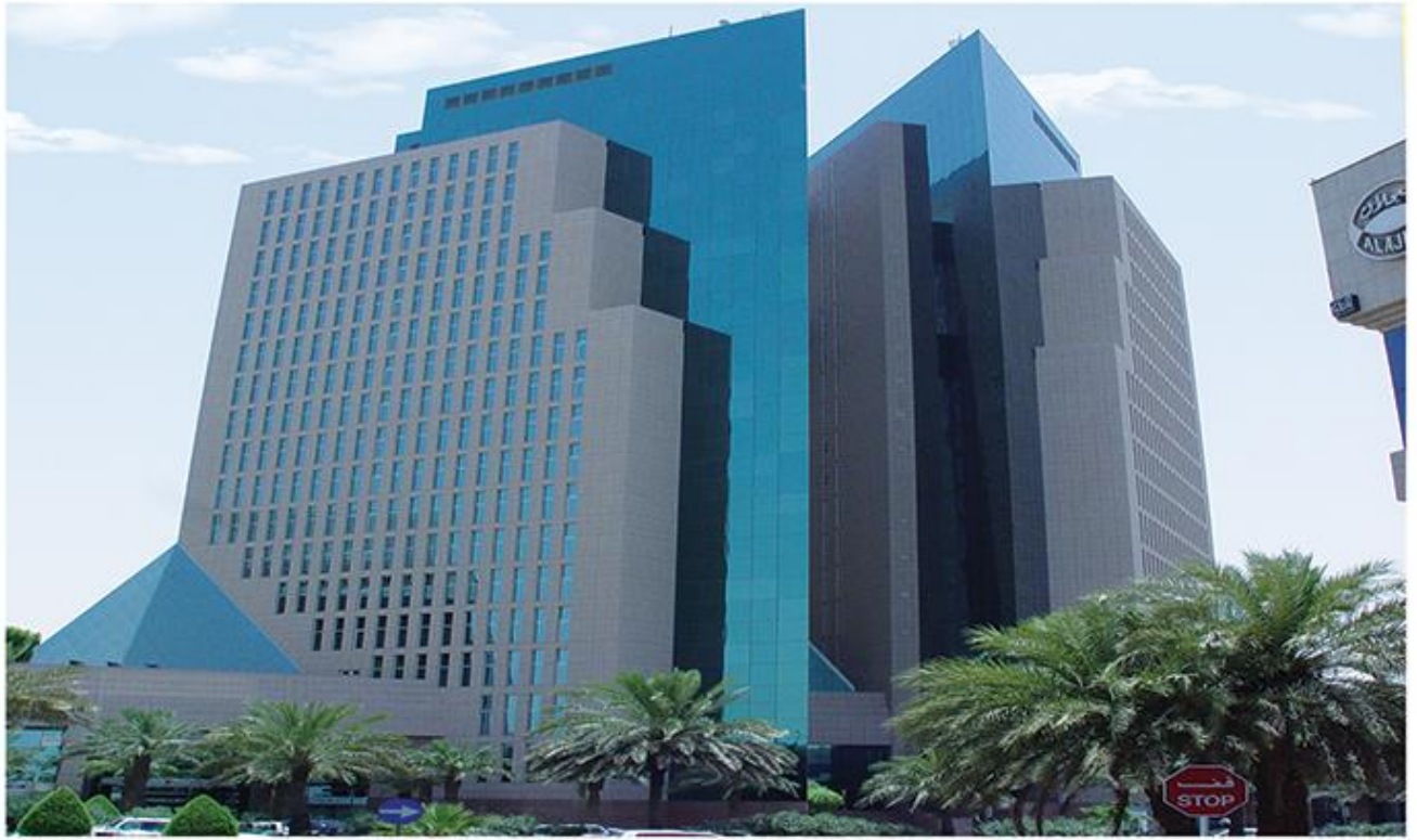
TAWINIA TOWER Waterproofing for bathroom by LM60
