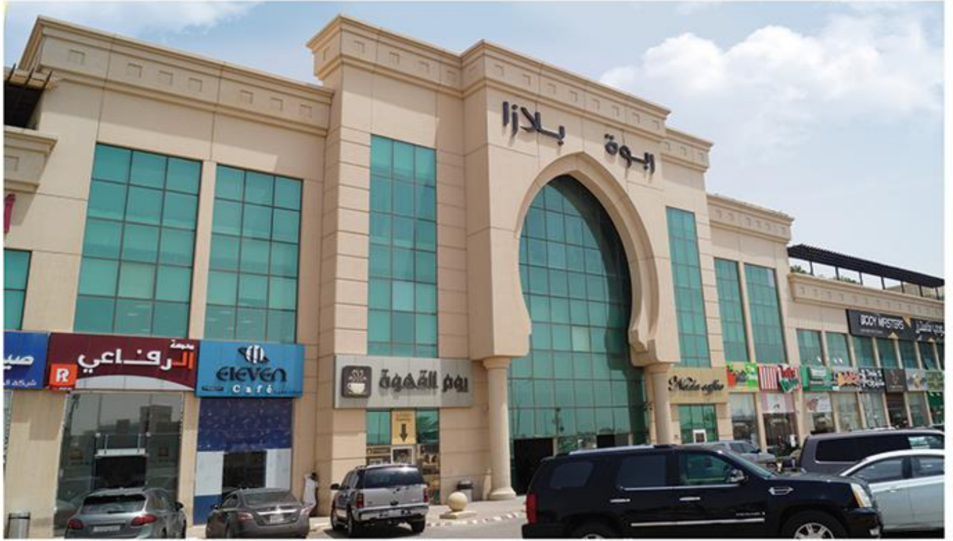
Rabwa Plaza Epoxy Works for Parking Area
