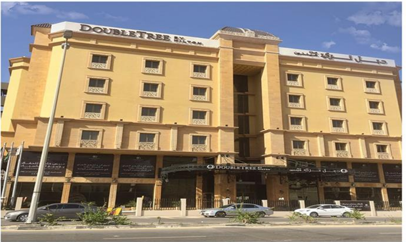
Double Tree by Hilton Hotel Thermal Insulation & Waterproofing
